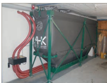
Abb. 12: Konussilo in Modulbauweise
